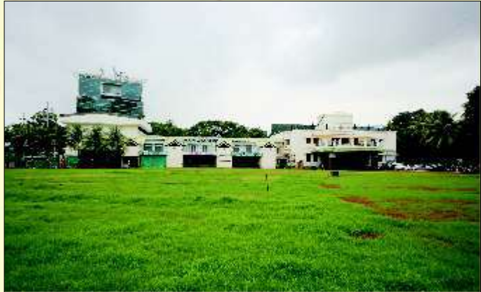
GYMKHANA VIEW FROM GROUND
