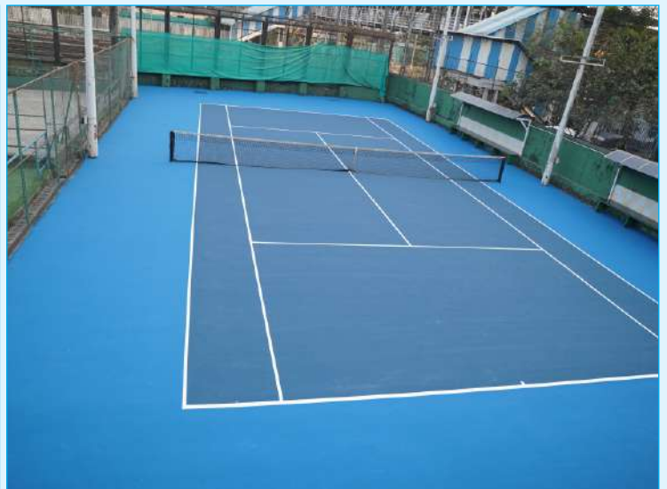
Resurfacing work of Lawn Tennis Court done by using Laykold Advantage (4 Layer Systems) • 1 x Primer • 1 x Black Base • 1 x Color Base • 1 x Top Finish • Line Marking
