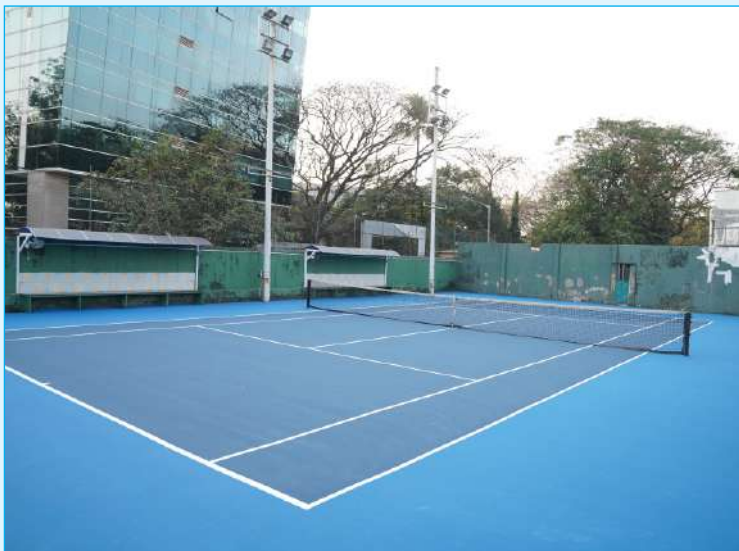
Resurfacing work of Lawn Tennis Court done by using Laykold Advantage (4 Layer Systems) • 1 x Primer • 1 x Black Base • 1 x Color Base • 1 x Top Finish • Line Marking
